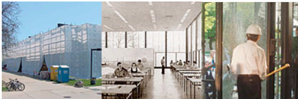
The contractor shrouded the entire building (1) to keep the dust from the lead-based paint from escaping into the environment. Students work at Mies-designed drafting tables in 1956 (2). Mies’s grandson, architect Dirk Lohan (3), ceremoniously launches the restoration by smashing one of the glass panels.
